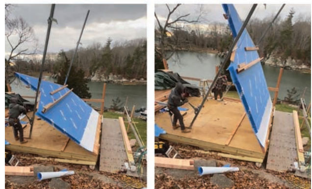
△ Figure 9. (top) Prefabricated NLT panels delivered to site by one person in a pickup truck; (bottom) two people tilt-up north gable wall. (Credit: Carbon Containment Lab, 2023)
