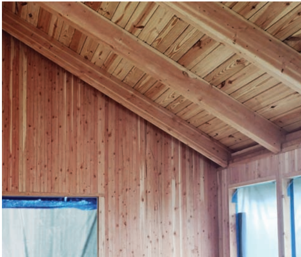
△ Figure 2. Hybrid wNLT and light wood framing on Demonstration Building, Guilford, Connecticut, 2024.
